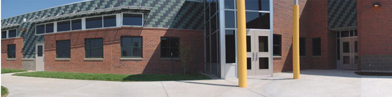
Figure 2: Front of Zach Elementary School, in Colorado where the TES optimal Controller is being implemented and tested
